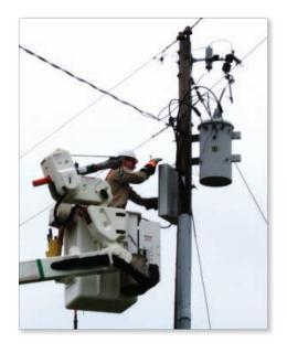
Multiple ENGO-V10 devices can be deployed along a feeder to provide fast voltage support and accurate control, with no fighting, along a feeder or the entire edge of a distribution grid network.
